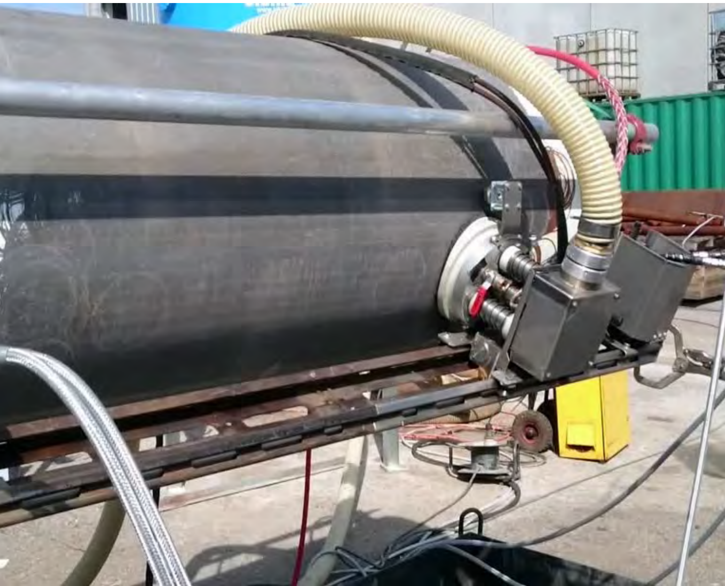
Nalta Jetframe 101, equipped with a rotor cradle and vacuum suction, used on a steel pipe for toxic paint removal.
